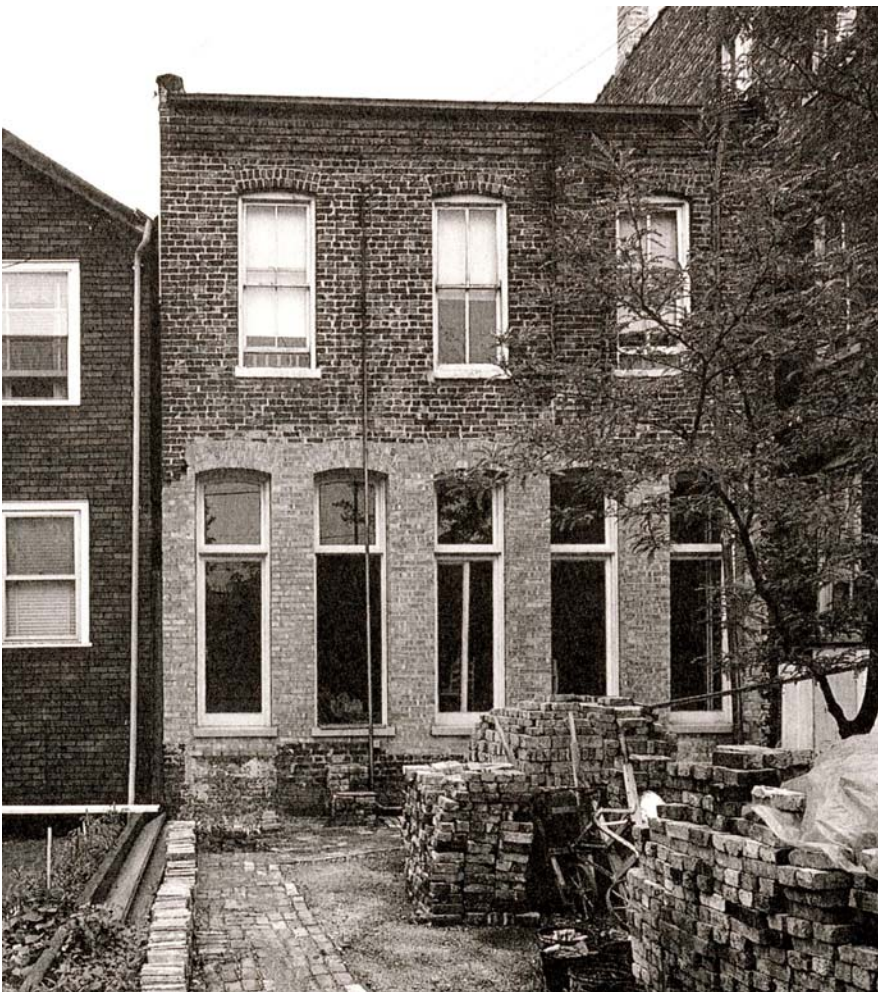
In February 1969, Richard Nickel purchased the two-story bakery and flat building at 1810 W. Cortland Street with the intention of gradually converting the building into his home and studio. Above: photograph taken by Nickel after he purchased the building. Left: the rear elevation of the building showing the reconstructed lower half of the rear wall.
